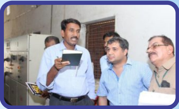
Shri. Ankush Bhartiya, Vice President inspecting the new cold storage unit
